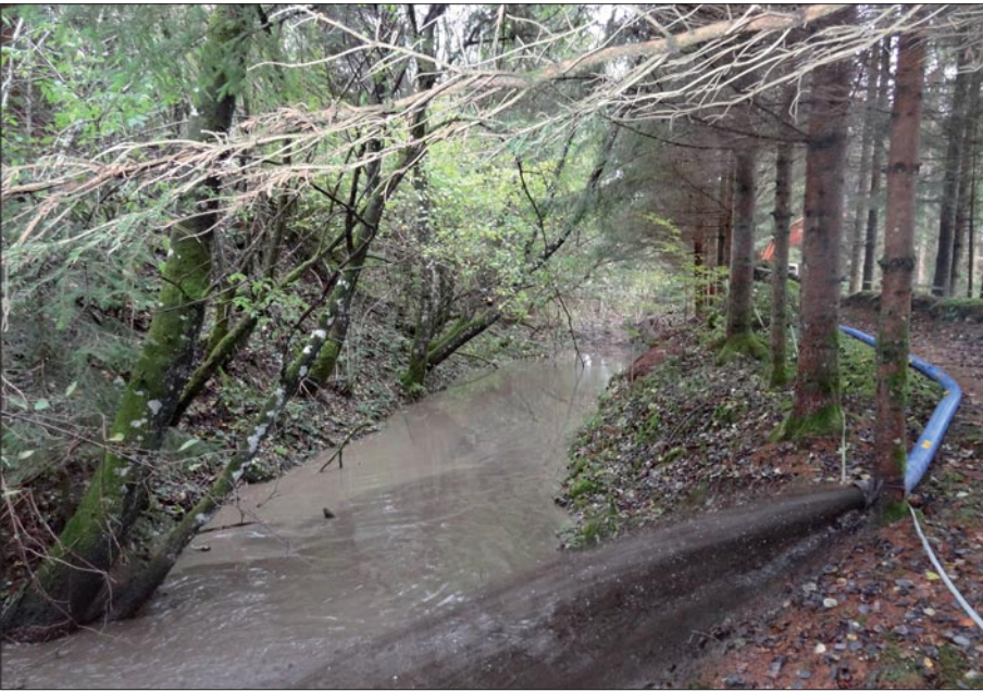
[6] Discharge of bottom deposits from Chailloux pond into settling ponds
