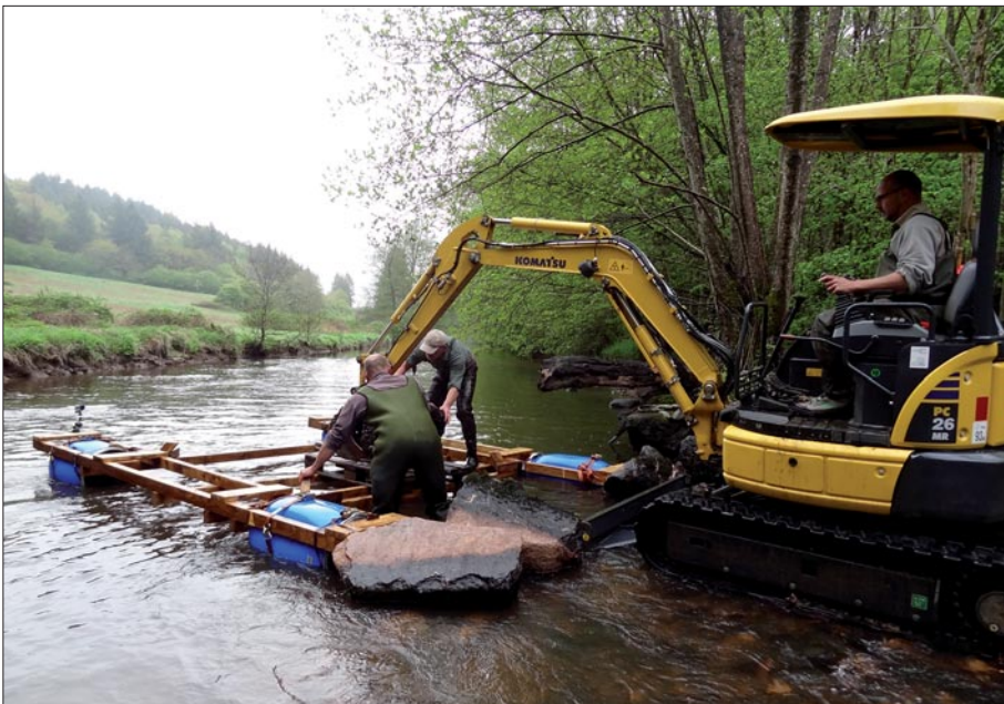
[4] Raft transport of granite blocks making up the Côte Cadoux sill
