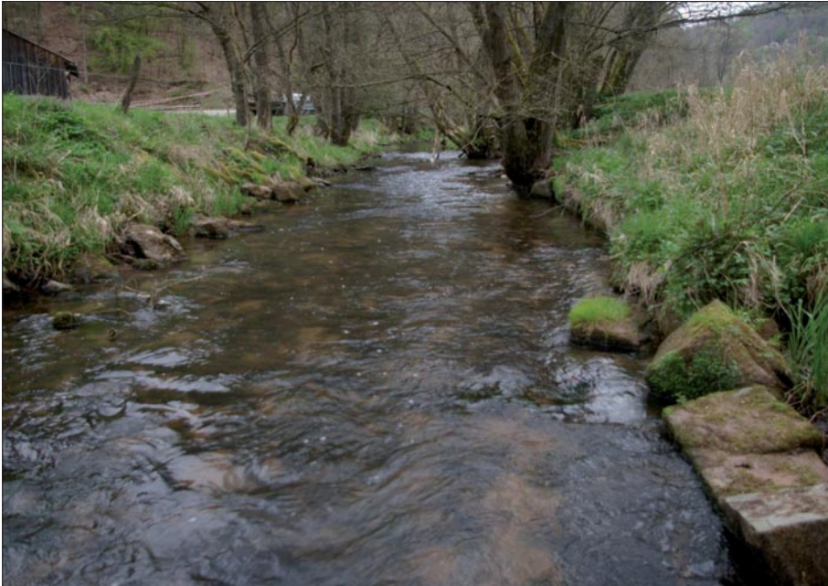
[7] Paved river banks result in the processes of a confined river zone.
