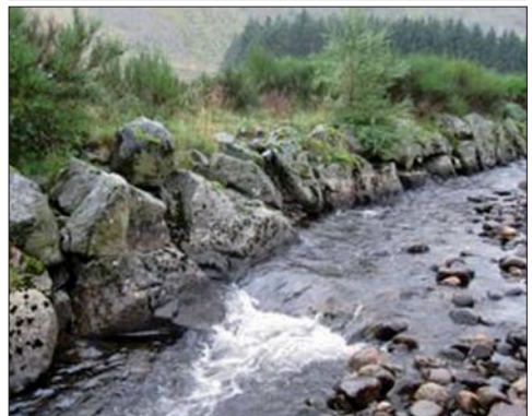
[2] Typical bank protection
