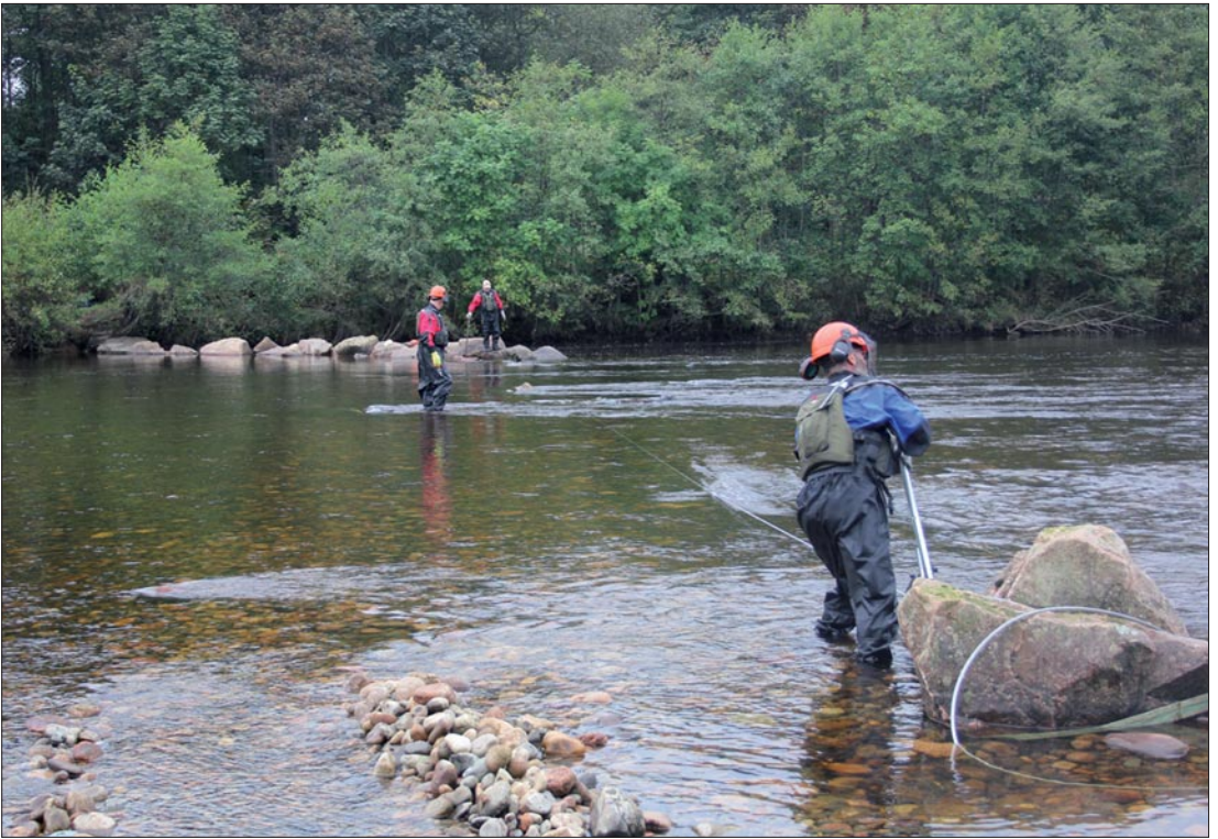
[3] Breaking up current deflectors using a hand-winch
