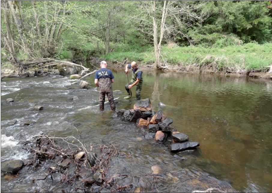
[3] Manual demolition of the Côte Cadoux sill
